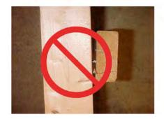
7. Use appropriate screws when attaching the stringer to a metal stud.
